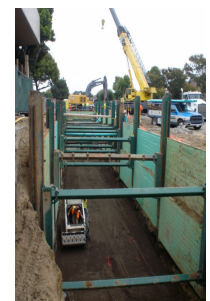
Hydraulic Trench Shield: very high clearance, 'MAXSHORES' .
