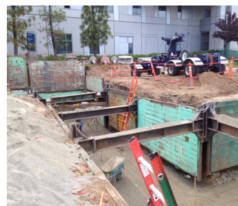
Hydraulic Trench Shield: very high clearance, 'MAXSHORES' .
