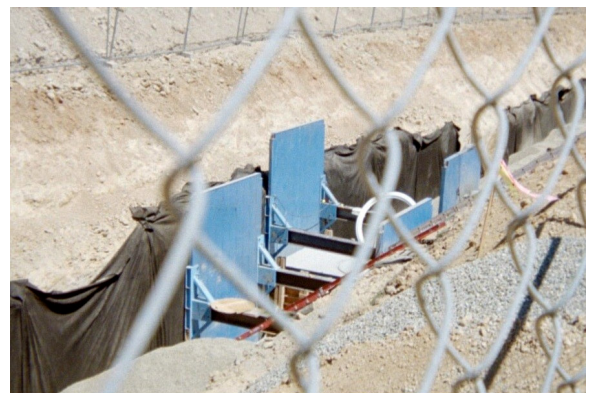
Hydraulic Trench Shield: very high clearance, 'MAXSHORES' .
