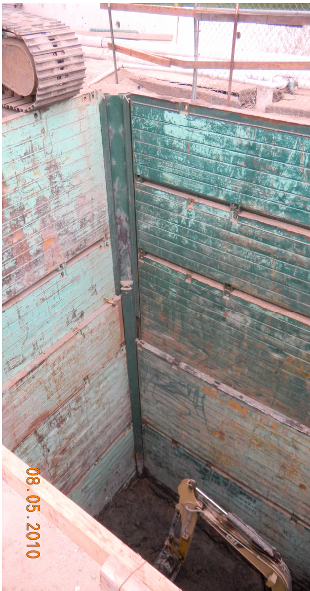
Telescopic Slide Rail Shoring: 35' Deep.
